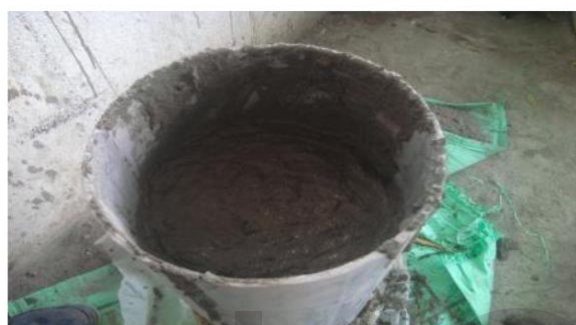
Figure 2: Casting of Column
