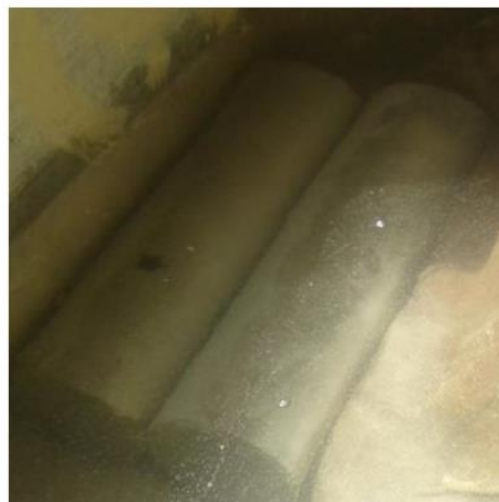
Figure 3: Curing of Column
